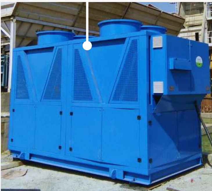
BATCHING PLANT CHILLERS
