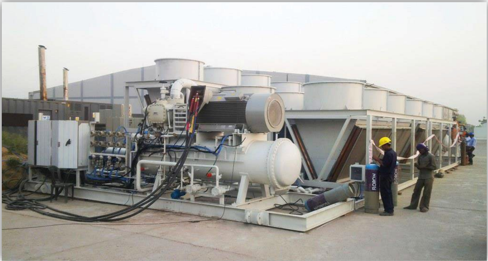
1000 TR, Air cooled, HT Motors, Installed at QChem, Qatar
