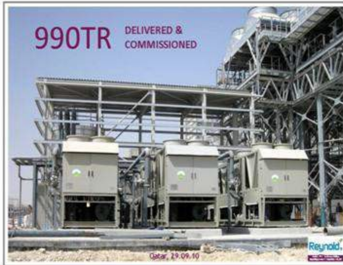
990 TR at Qatar for process cooling
